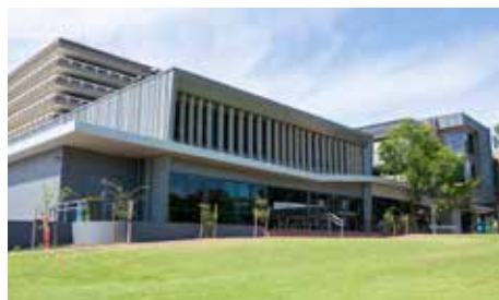
Wirrkuta Trruku is an activity hall with a gym, chapel and dedicated OSHC facilities.
