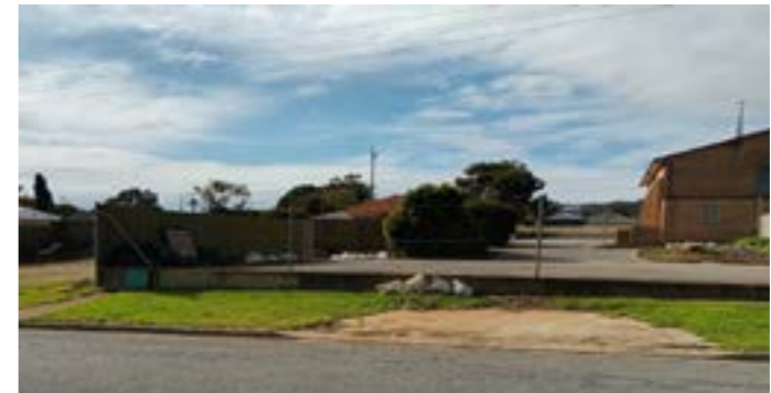
The unused piece of church land (above) before it was transformed into purpose-built homes for LDS clients (right).
